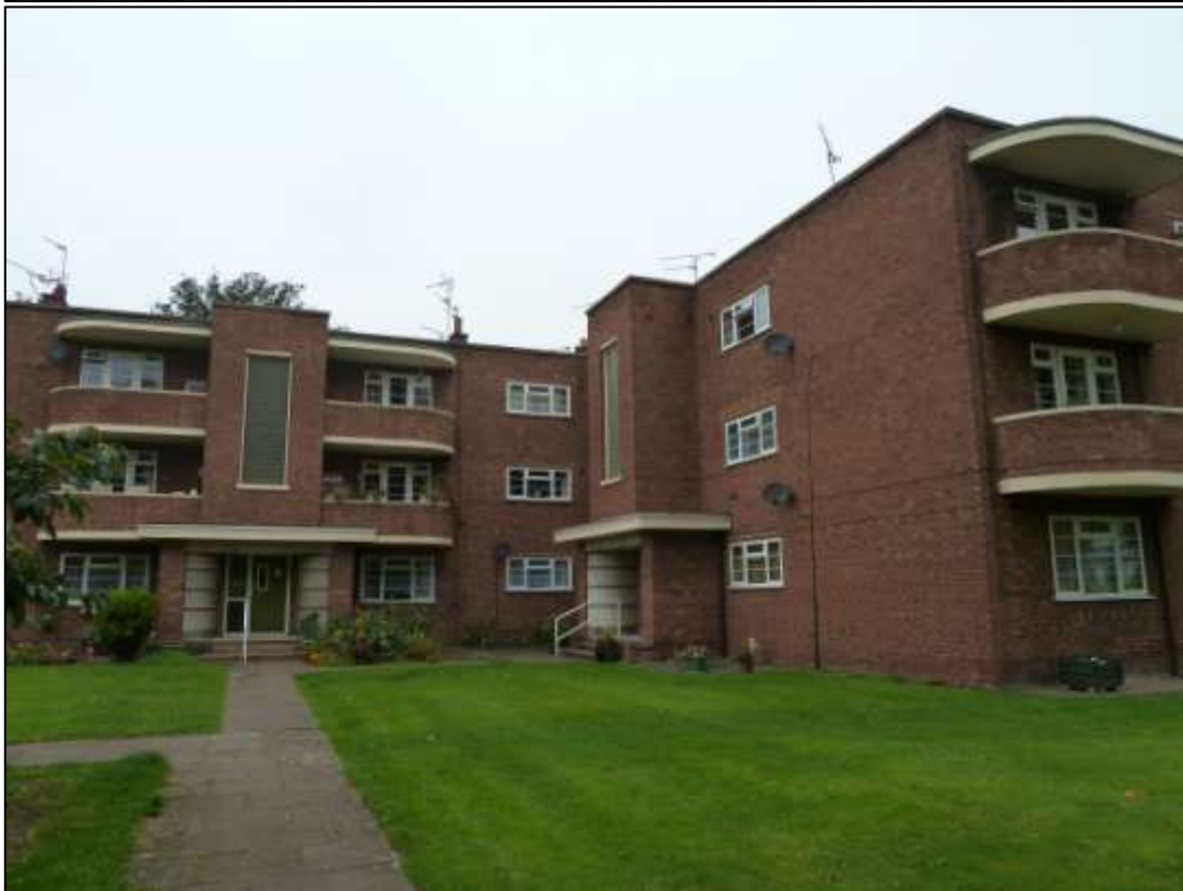
Figure 8 Corporation Street flats from Corporation Street
