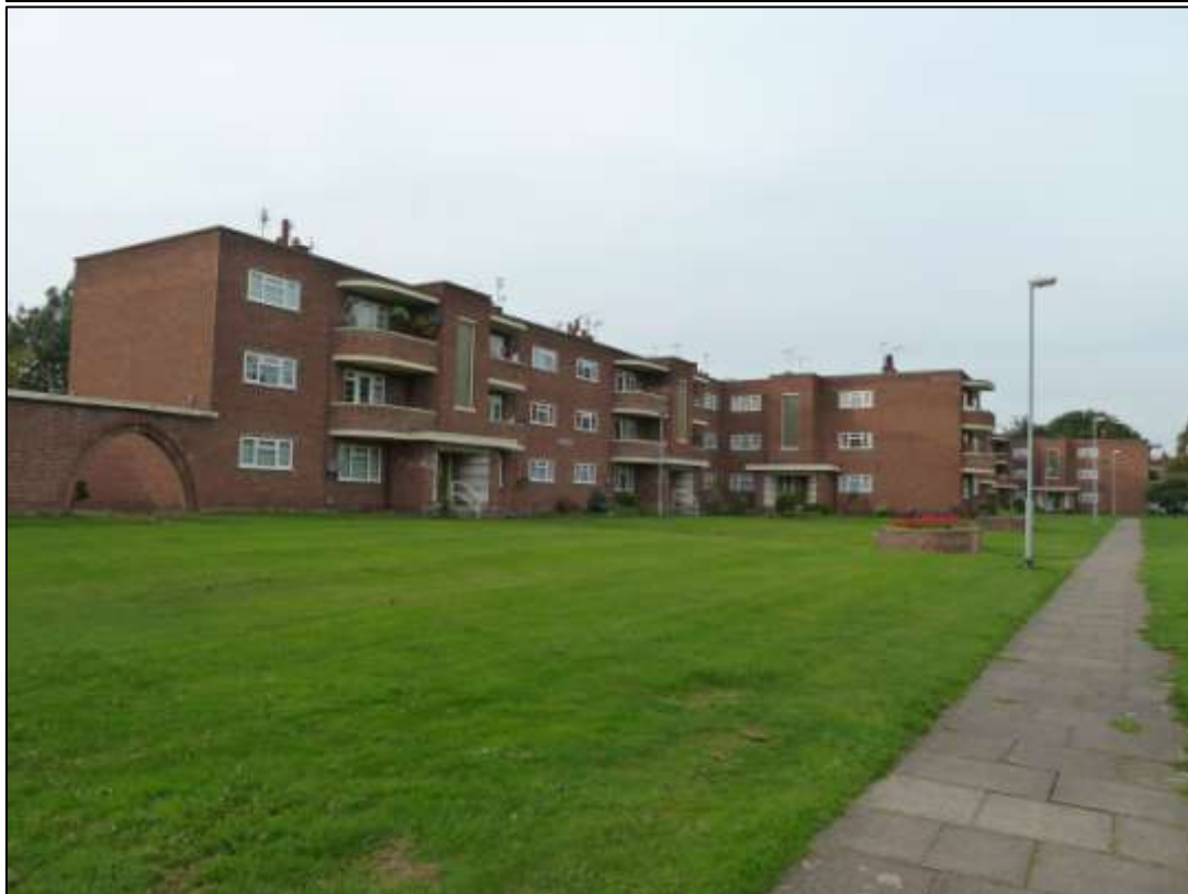
Figure 9 The green space and trees create an inviting setting for the flats and reflect Modernist municipal housing principles
